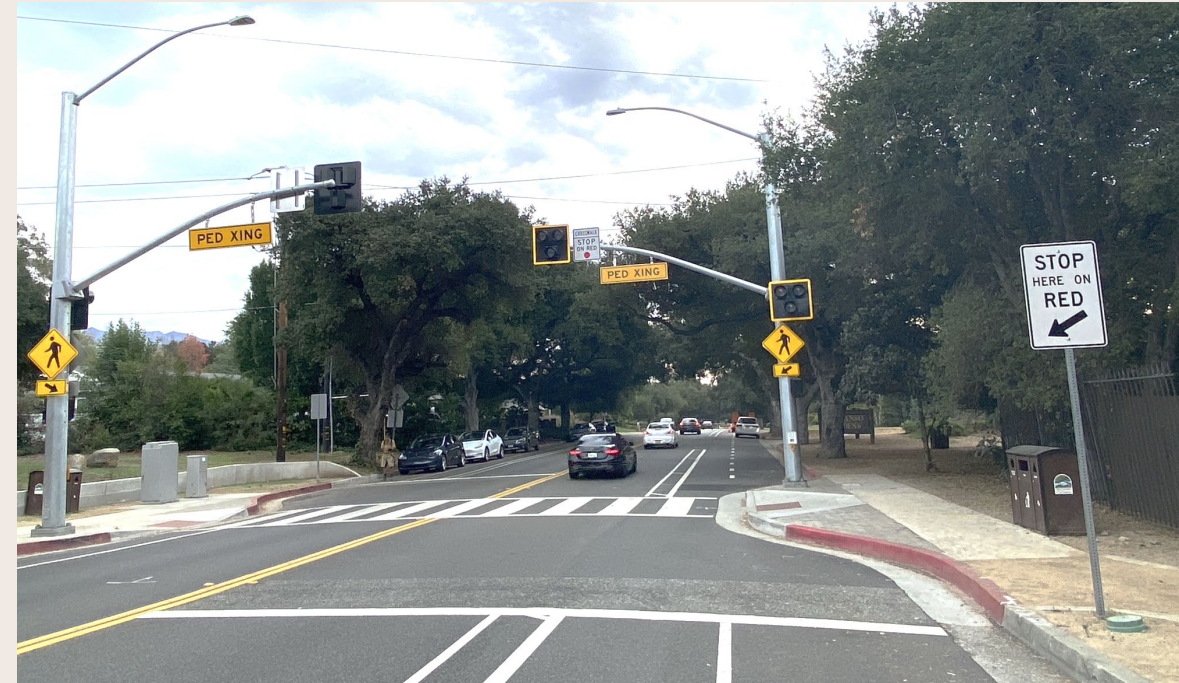
Descanso at Trail Crossing High-Intensity Activated Crosswalk (HAWK)
