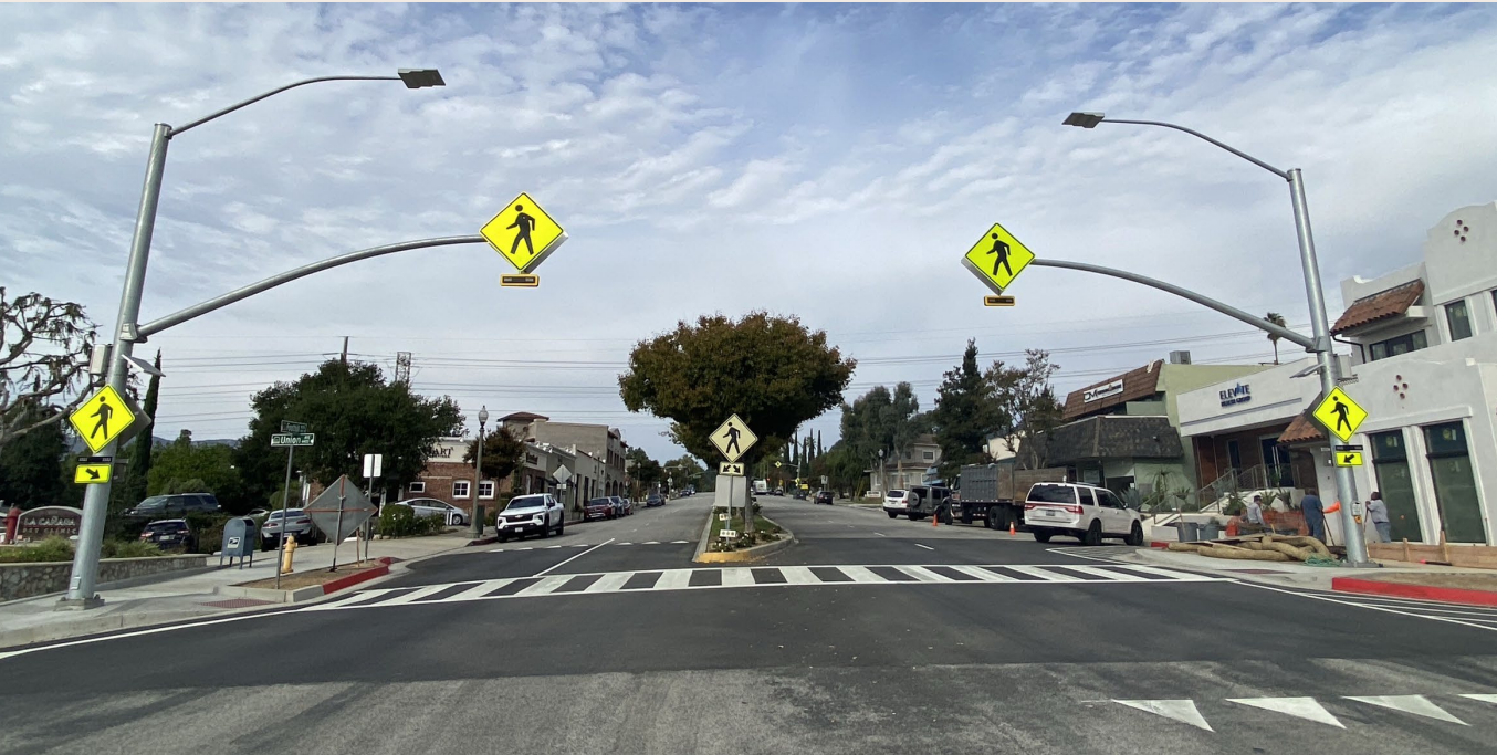
Foothill at Union Rectangular Rapid Flashing Beacon (RRFB)
