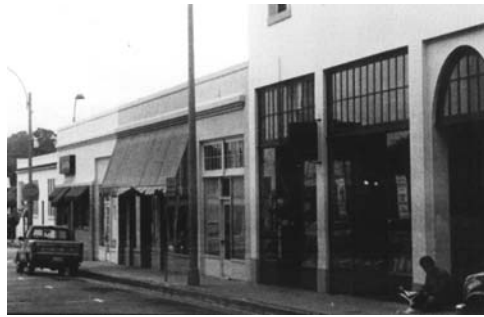
Higher glazed areas are appropriately used in the larger building. The use of transom windows makes the interior more pleasant while making the exterior more inviting and better proportioned.
