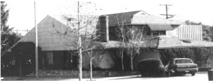
This longstanding commercial building features complex roof forms more commonly seen on residential structures.
