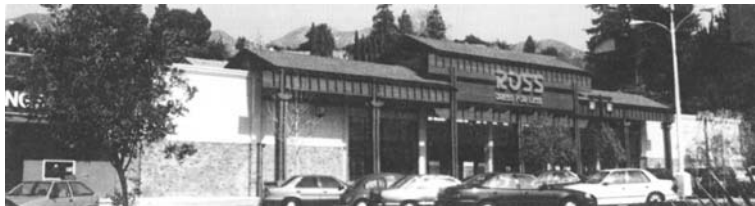
The use of pitched roofs visibly fronting and extending back over the vast and invisible main roof, are effective in bringing an inviting appearance to a converted supermarket.
